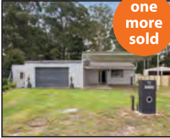
71 Waratah Crescent, Sanctuary Point
